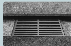
Storm Water Drainage
